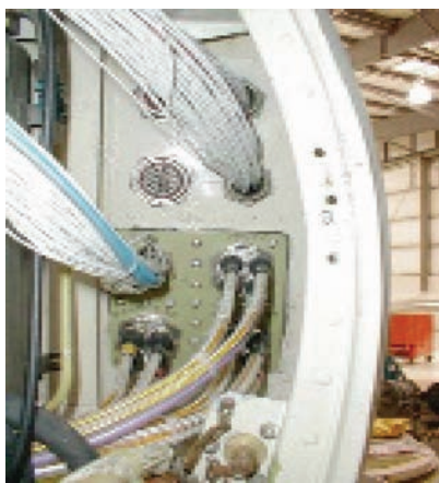
Installed QUAD Connector
