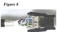
trim wires flush
