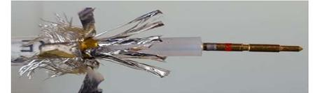
Figure 5 Install connector body &amp; trim to shoulder
